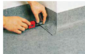
Trimming overlapping strip.
