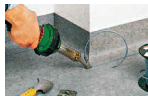
Sealing with weld rod.
