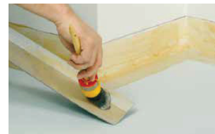
Apply contact adhesive up to the markings on floor and wall.
