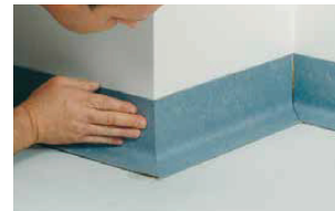
Fix cut-to-measure HSLA skirting in place.
