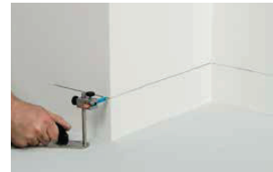
Mark walls for positioning of product.
